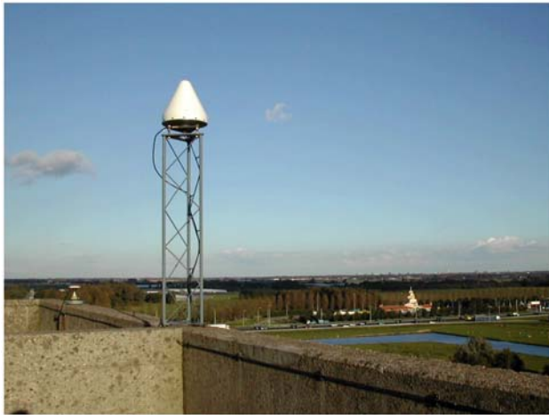
Figure 1: The Ashtech choke-ring antenna, with conical radome, installed on the observation platform of the (formerly) TU Delft building for Geodesy, for the static test. This site, about 30 meters above ground level, offers unobstructed visibility of the sky, down to the horizon. The satellite elevation cut-off angle was maintained at 10 degrees during the measurements (elevation cut-off angle for the data processing was 15 degrees).
